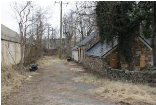
The Stone Bridge Tollhouse in 2009.
